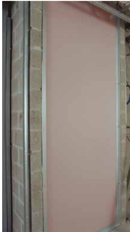
Figure 6: First Layer of Gyprock Fyrcek and Perimeter Framing Fixed
