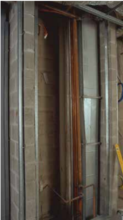
Figure 5: Service Shaft with Perimeter Angle Frame Fixed
