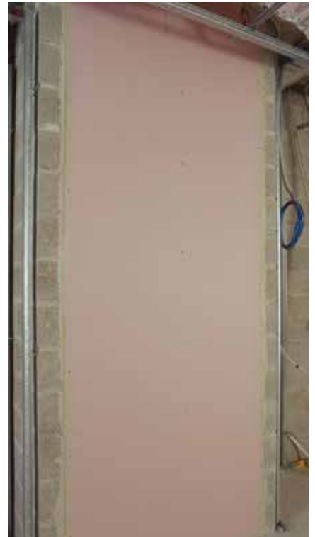
Figure 7: Gyprock Laminated Service System after Completion
